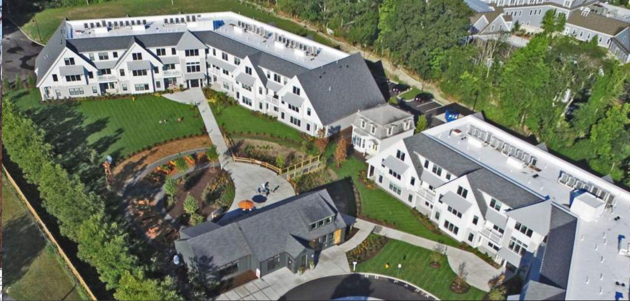
Oriole Landing | Lincoln, MA | 2020 | 60 Units | 72,000 SF
